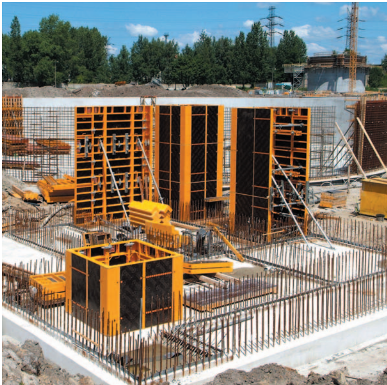
Construction of sewage-treatment plant in Katowice
